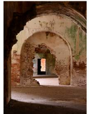
Clay Thurston of Knoxville, TN Fort Morgan Archways
